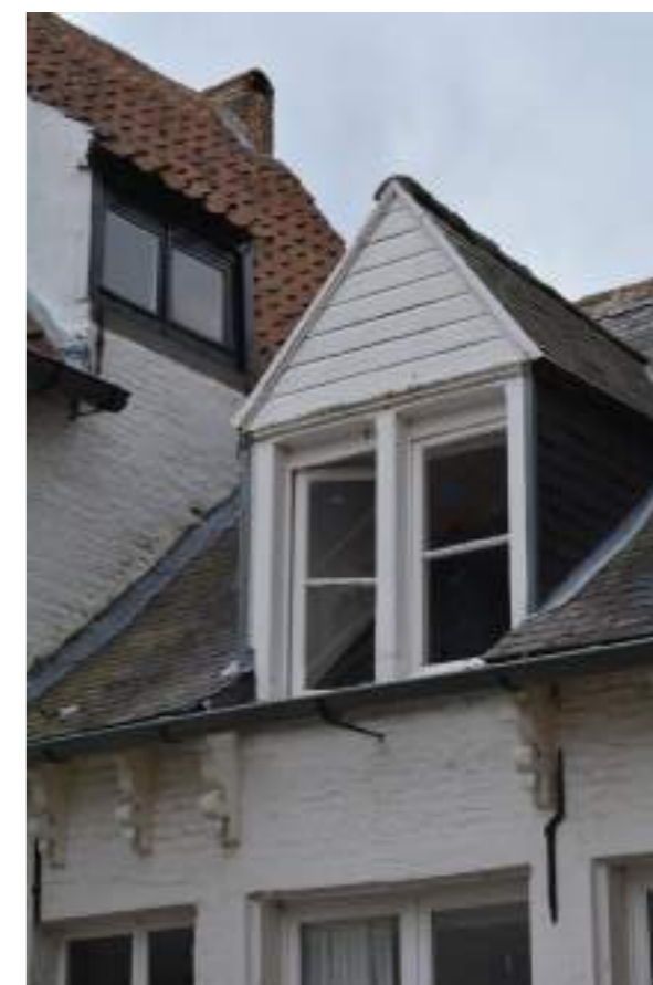
Fig.05. Detail houten dakkapel
